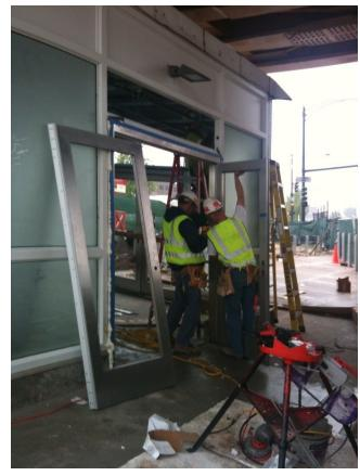
Archer stationhouse having final pieces of equipment installed including doors, lights, CA booth, and fare control equipment.
