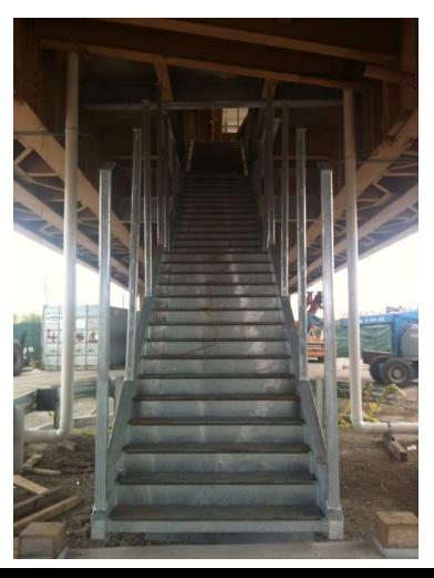
Structural steel in place for new staircase to platform and walkway to stationhouse.
